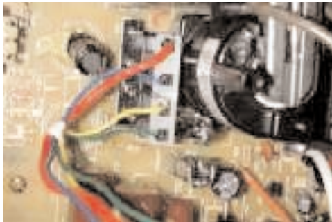
Original Yoke Wiring
